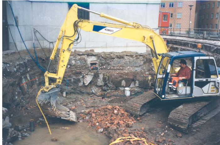
Close to the walls of the Parliament. Great forces are required when the 7 m long pole are pulled out of the ground.
