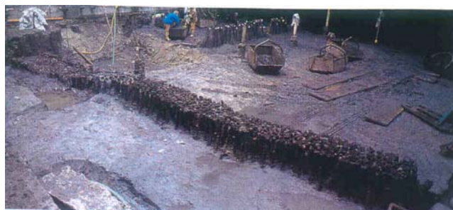
Figure 53a: The oldest foundation piles found recently within the basement of the building of the ex-cinema San Marco .
