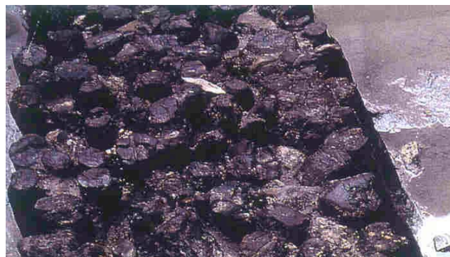
Figure 53b: The row of piles is made of small logs 8 to 16 cm width.
