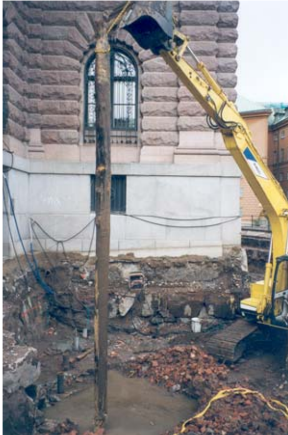
Two poles are pulled out the ground after 113 years of service. Note the stone foundation and the old backfilling, -a blend of bricks.
