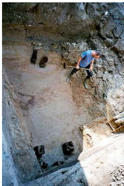
Figure 2. Overview of the excavation pit. Two piles can be seen at the west side of the pit (top of picture), four on the east side (bottom of picture). Of the latter, three were sampled for BACPOLES. Directly to the left of these piles, the small sandy plateau is the location of an oil tank.
