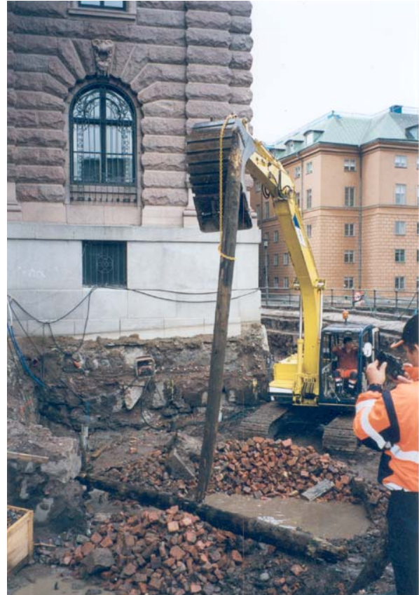
Two poles are pulled out the ground after 113 years of service. Note the stone foundation and the old backfilling, -a blend of bricks.
