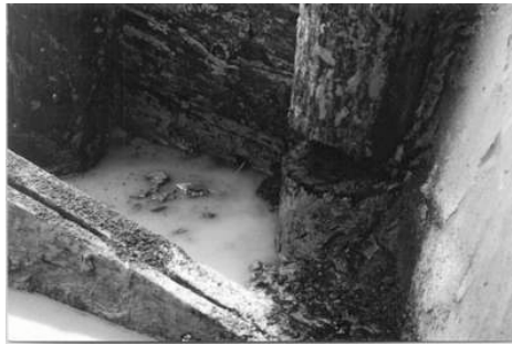
Figure 7 Oak pole of the embankment after the woodsample ("wedge") had been taken
