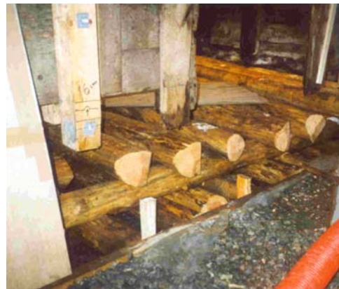
Pictures 2 and 3 reconstruction of the foundation in building Ve, in a traditional way with round wood Pine. The wood is covert salt crystal.
