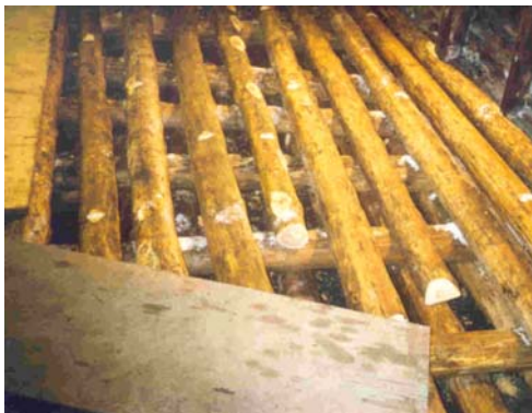
Pictures 2 and 3 reconstruction of the foundation in building Ve, in a traditional way with round wood Pine. The wood is covert salt crystal.
