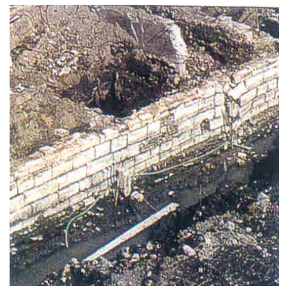
Figure 56c: The long wall of Istrian stones, with its foundation piles beneath, dating 16 th century, found on the island of Giudecca .
