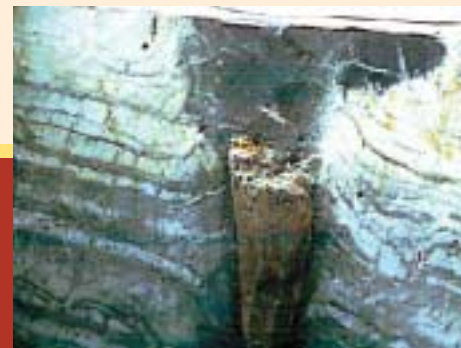
Medieval foundation pile in sandy soil. Most of it has disappeared because of degradation processes in the soil.
