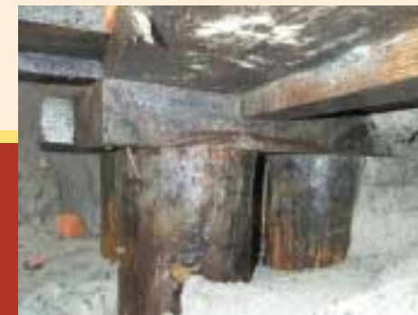
Excavated foundation piles in Amsterdam.
