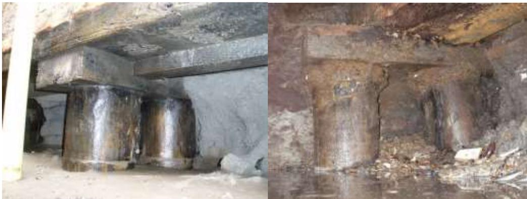
Figure 10. Two examples of common Dutch foundation constructions: two piles connected by a beam, covert by horizontal planks on which the bricks are situated. Both planks and beams are loaded perpendicular to the grain.
