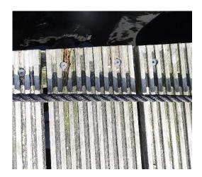
Landing stage 13 gangs boards of several species (manbarklak, angelim pedra, aldina, faveira amargosa), horizontal construction beams based on the goms flecks identified as angelim pedra, and the acariquara pole with the original tree trunk shape (non-machinable, e.g. non sawn). The condition of gang boards, horizontal construction beams and pole is good.
