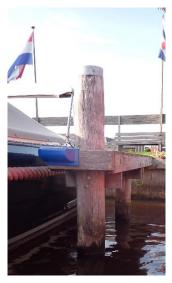
Sign with landing stage seven turns out to be incorrect. The gang boards are made of bamboo and not of tanimbuca (= gindya udu), and the horizontal construction of angelim vermelho.
