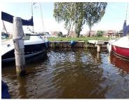
Sheet piles 11, azobé, sheets are a supposed continuation of the reused azobé under 9 until the corner of the island. Thickness 40 mm. Some plants grow through the seams, wall is coherent. Condition questionable (visual / awl waterside hard, landside not reachable, density profiles show moderate decay in upper part and in lower parts weak decay land- and waterside 5-10 mm; the same sheet pile is sampled (M14) as from which the density profiles were made, is the last pile of this species.
